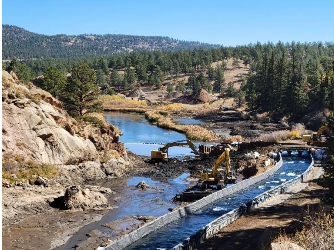
Lake George diversion dam removal
