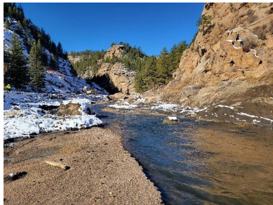
Lake George diversion dam after removal
