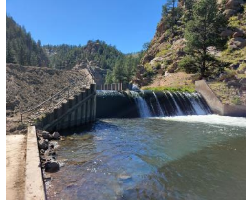
Lake George diversion dam before removal
