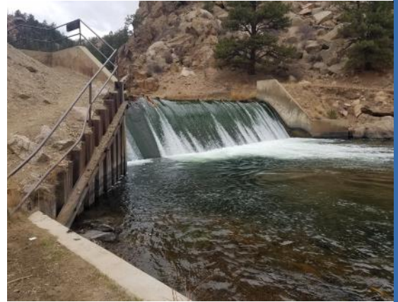
Lake George diversion dam removal
